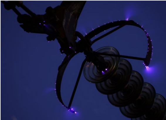
Figure 2: A corona discharge on an insulator string of a 500 kV overhead power line. Image by Nitromethane , own work, CC BY-SA 3.0
